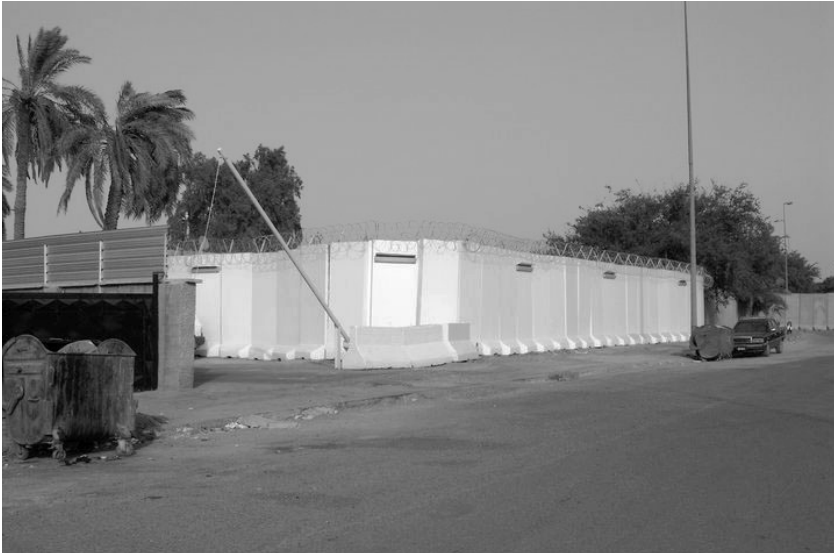
Figure 17.2. TONI compound's walls. View from inside the International Zone, Baghdad, 2010
