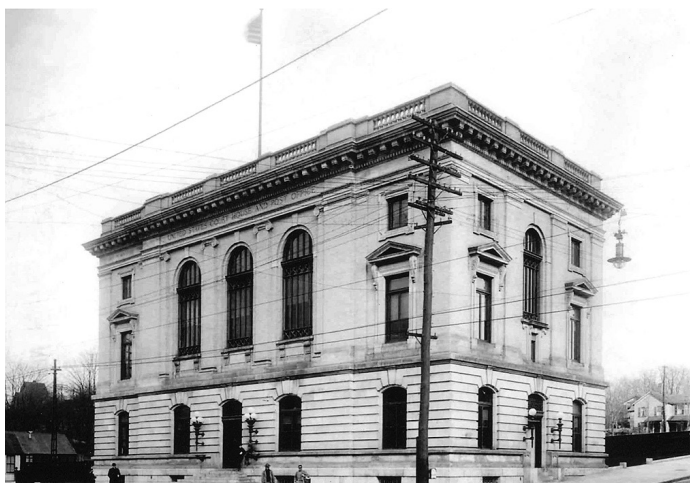
Figure 1.10. The 1904 Court House and Post Office at the corner of West 3 rd and Washington Streets—demolished in 1962. (Fenton History Center)
